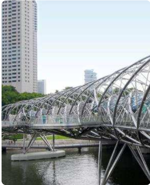
Marina Bay Bridge, Singapore
